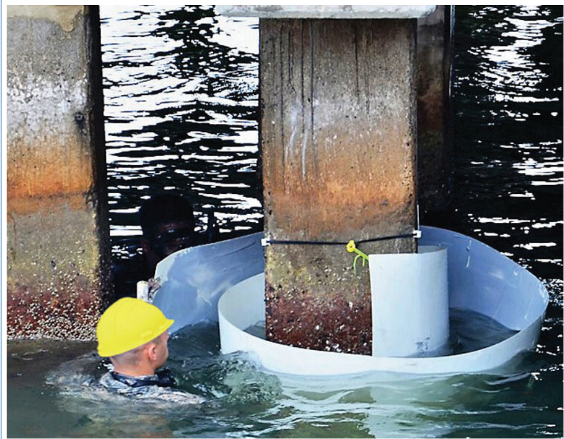
Photo 3-21: Glass fibre reinforced polymer jacketing
