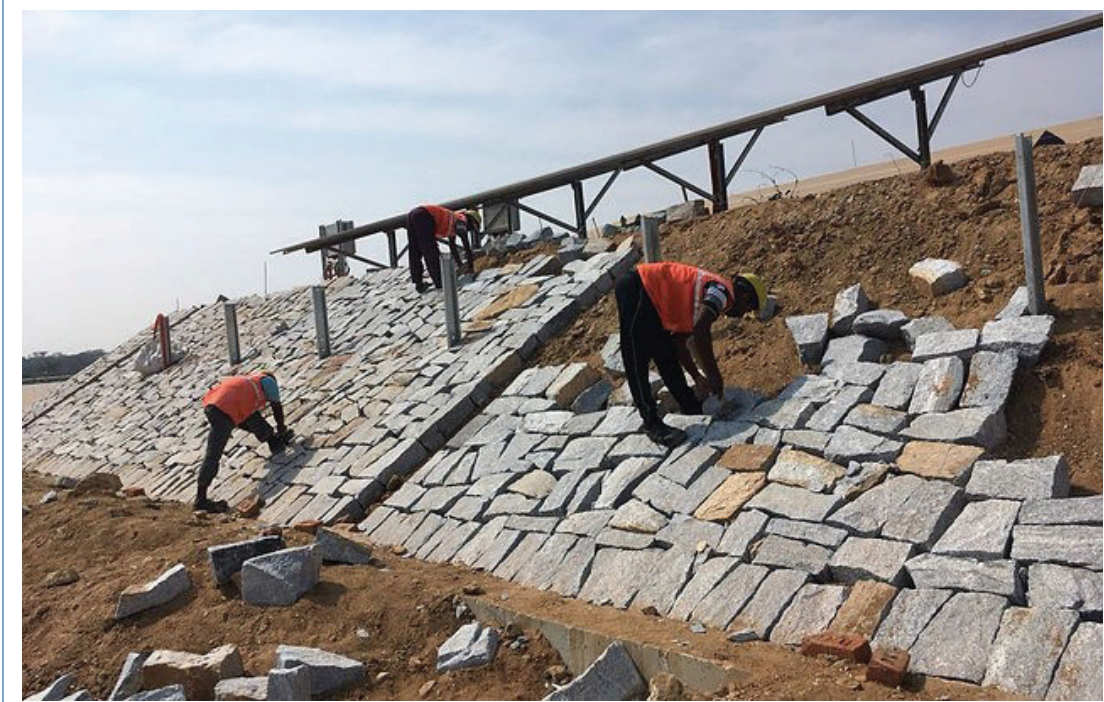
Photo 3-22: Laying of stone pitching
