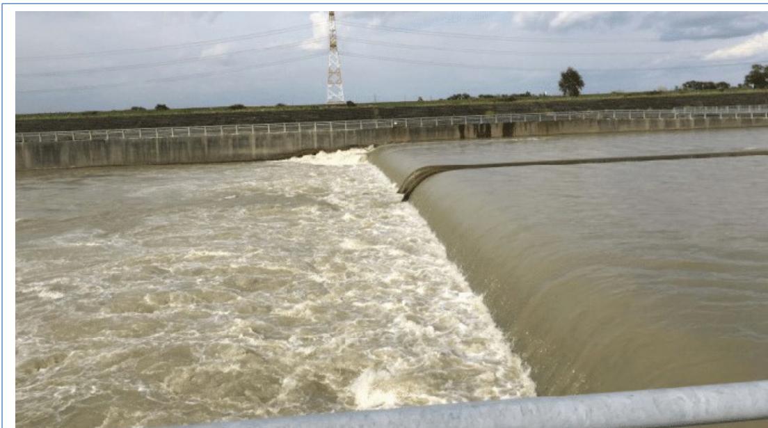
Photo 3-23: Side elevation of a weir
