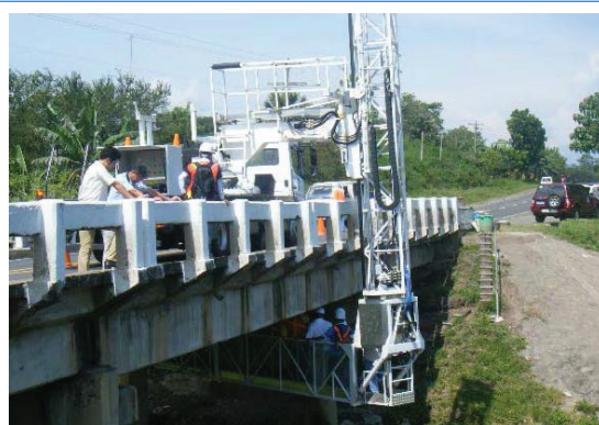
Cleaning using inspection vehicle
