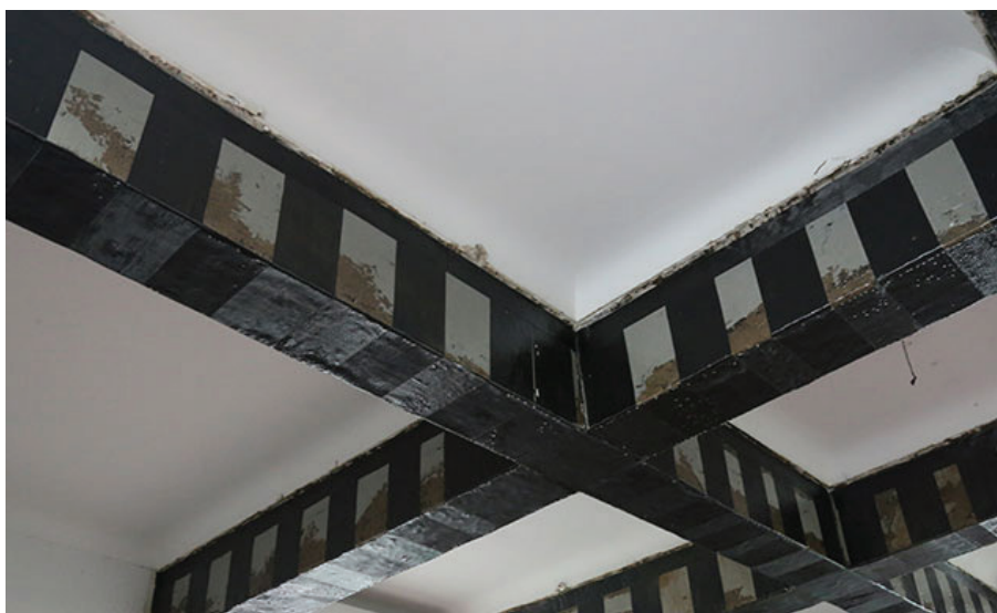
Photo 3-20: Fibre reinforced polymer jacketing
