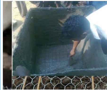
Ferro-cement Method of Repair
