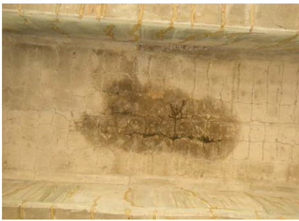
Photo 3-1: Severely Damaged Deck Slab
