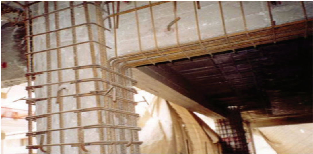
Photo 3-18: Reinforced concrete jacketing
