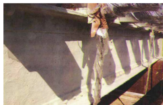
After completed 2 nd layer painting
