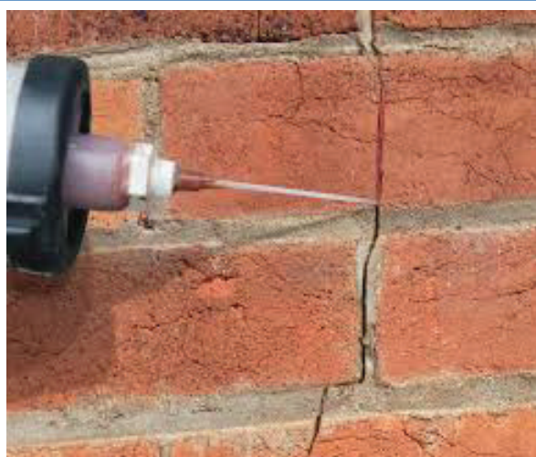
Epoxy Resin Injection
