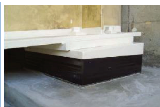
Photo 3-13: Sample of replacement of bridge bearing
