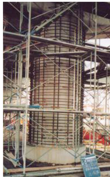
Concrete Jacket for Pier Repair
