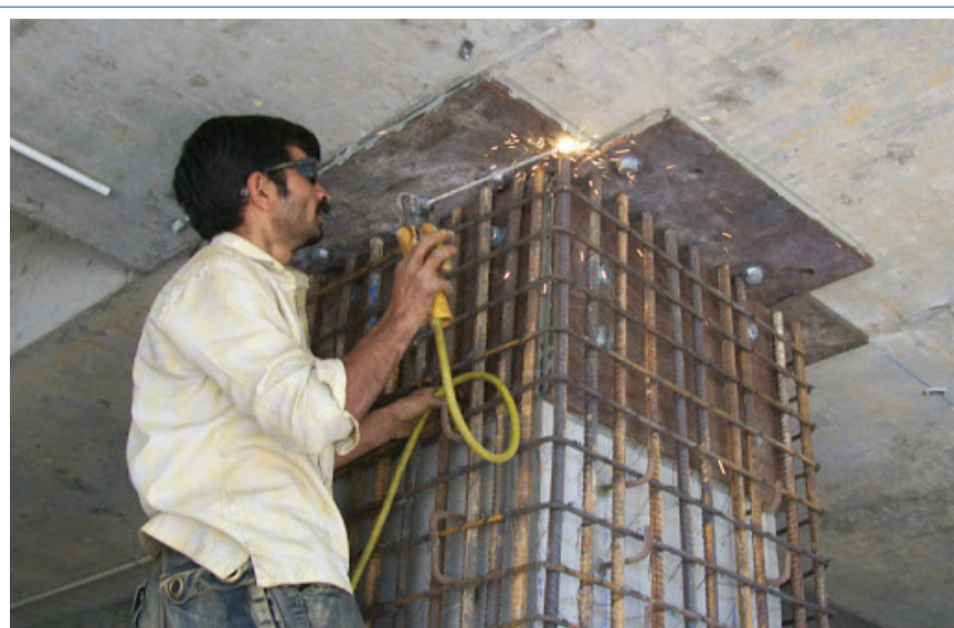
Photo 3-17: Welding of reinforcement bars
