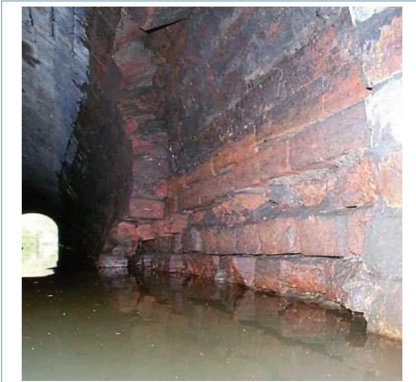
Photo 3-8: Missing block
